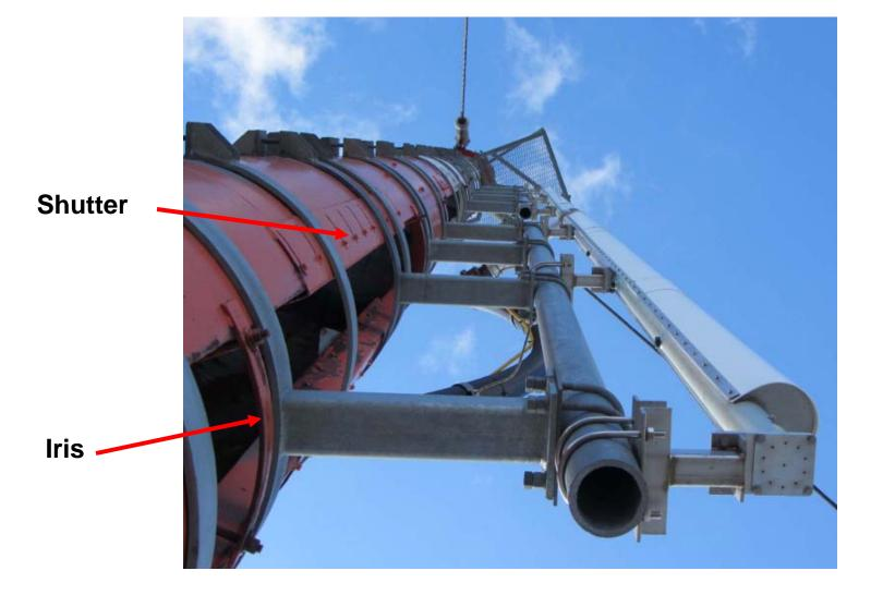
The picture above is a of a new Omnioid channel 42 antenna outrigged on an old channel 5 Omnioid slot antenna (left in orange). The channel 42 antenna pylon is 3-1/2 inches (8.9 cm), while the old channel 5 antenna is 4 feet (122 cm) in diameter.
